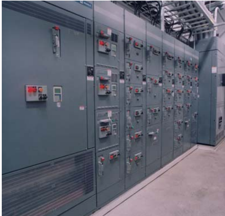
Intelligent motor control center
