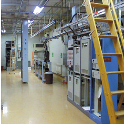
Telephone Switch Room
