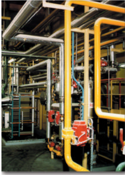
Piping System for Liquid Process Ingredients
