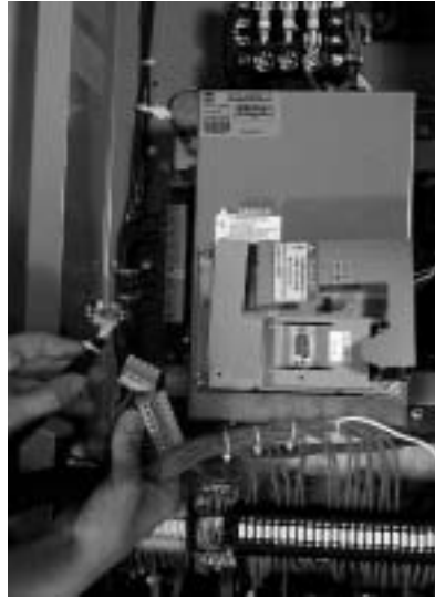
Figure 21: Remove All Power and Control Wiring
