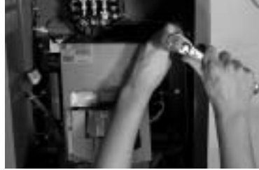
Figure 22: Remove Picture Frame Screws
