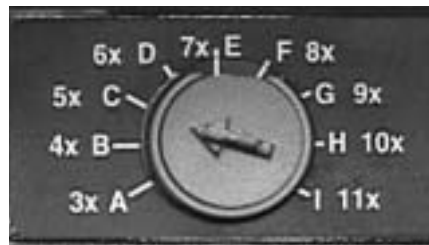
Figure 15: Circuit Breaker Trip Adjustment Dial
