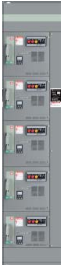
8998 ATV58 MCC Panel Section.tif
